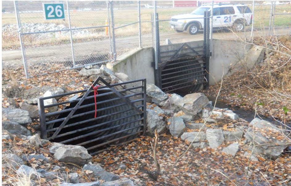
Figure 5: Existing Trash Racks North End of Mill Creek
